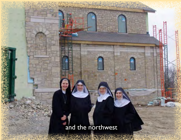
Progress on the southwest
