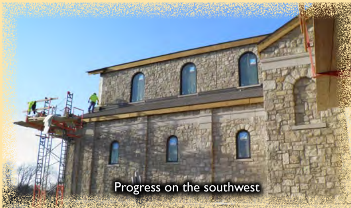
Work on the sanctuary groin vault
