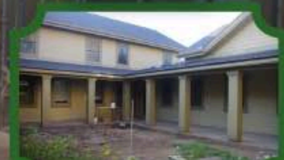
The nearly completed cloister
